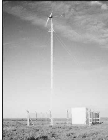
Hybrid Wind/PV system in Portugal
