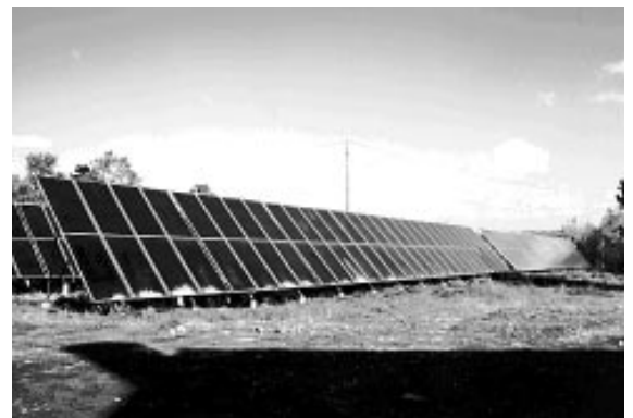
Mount Saint Vincent Motherhouse Halifax, Nova Scotia, Canada 224 G32 solar collectors 675 m 2
